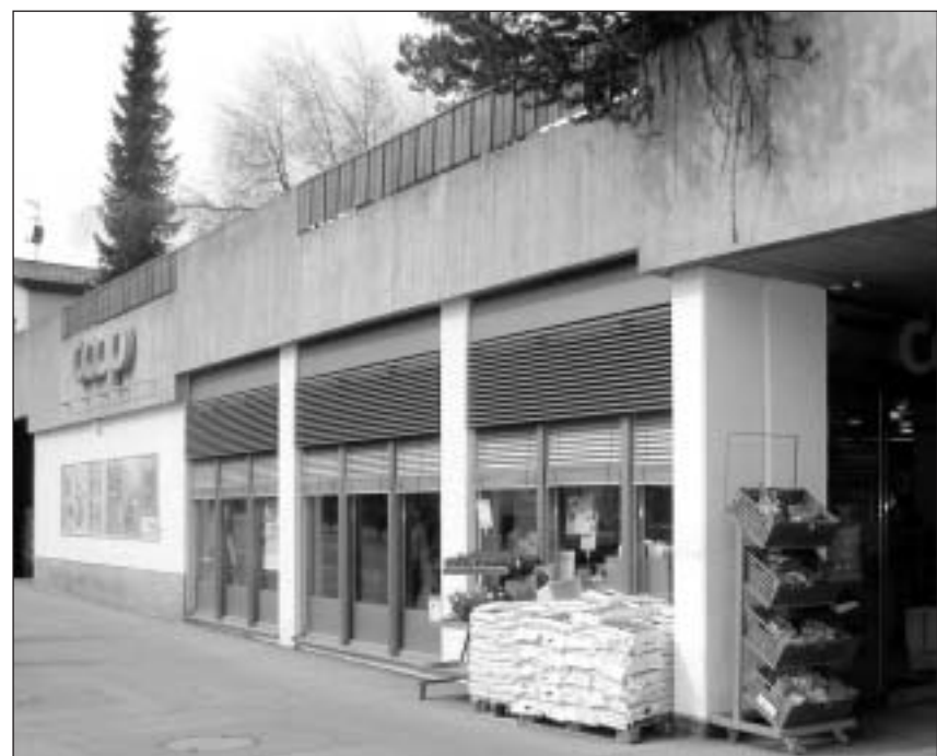
La stizun dil Coop a Mustér vegn renovada proximamein. Per quei intent sto ella vegnir serrada duront rodund in meins.
